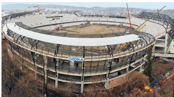
2011 - The "Cluj Arena" stadium under construction, preparing for this year's inauguration.
